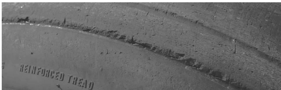
Figure 527. Groove Edge Chunking
